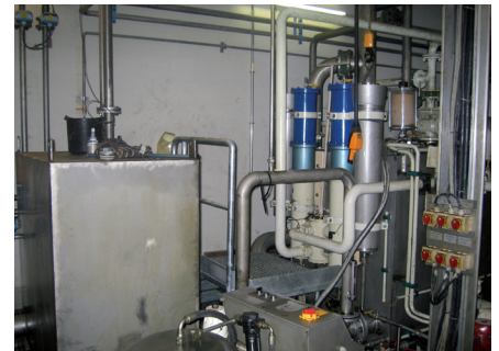
Lubricating oil circuit
